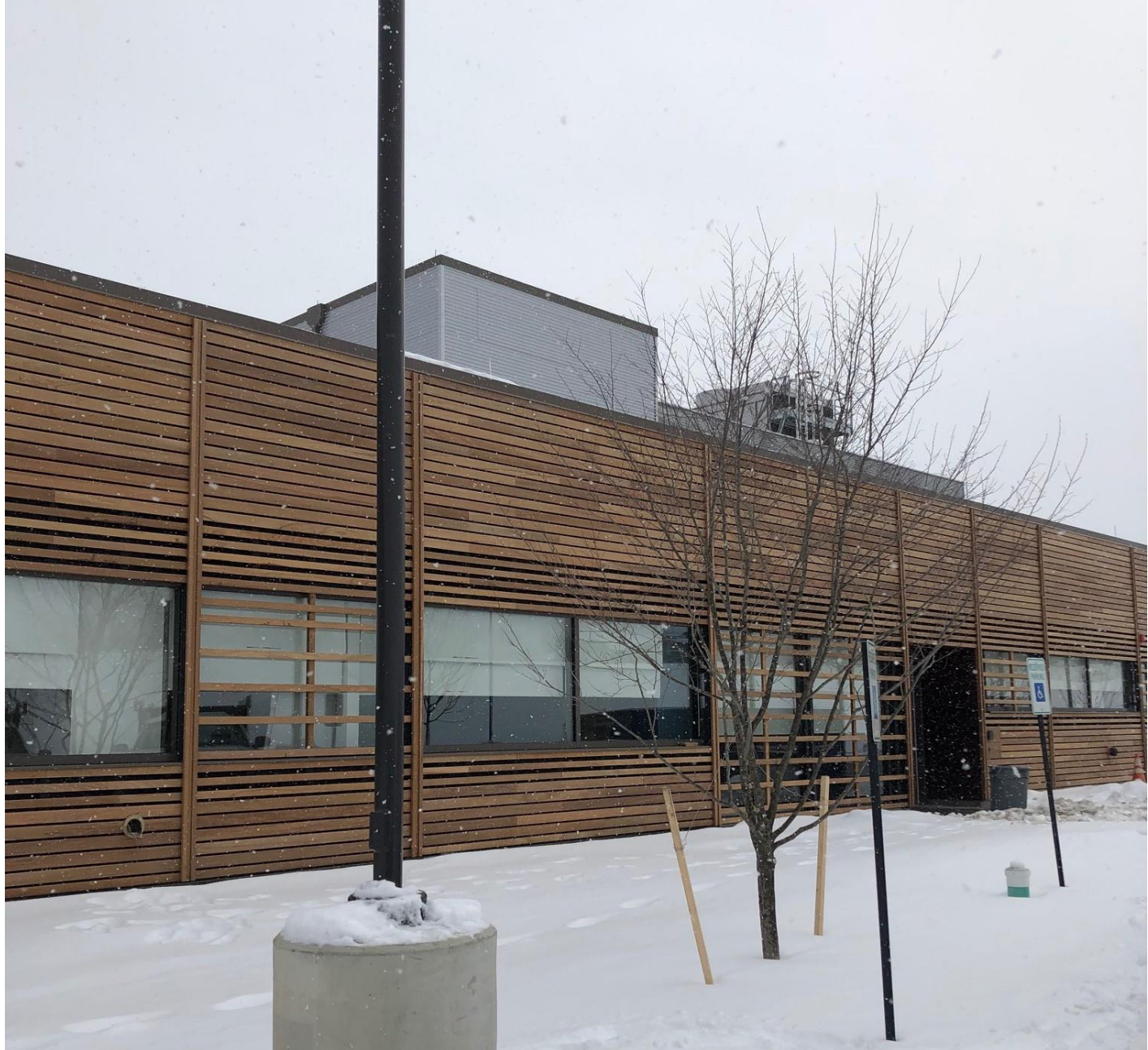
View of Office/Entry
