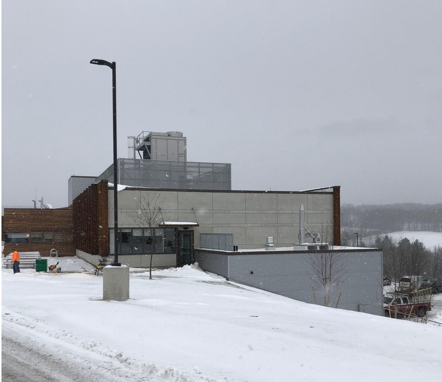
From Entry Looking North 10
